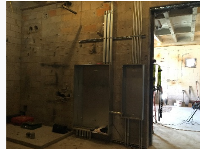
Installation of Electrical Main Panels
