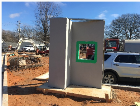
Mock Up Waterproofed & Prepared for Skin Components
