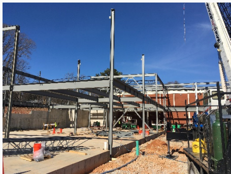
Installation of structural steel
