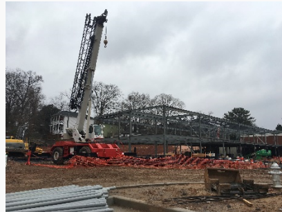
Structural Steel Erection
